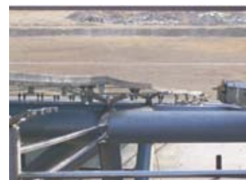
Cubierta sede central ZFP ZFP Headquarter's Skylight Jeddah, Arabia Saudi 2008
